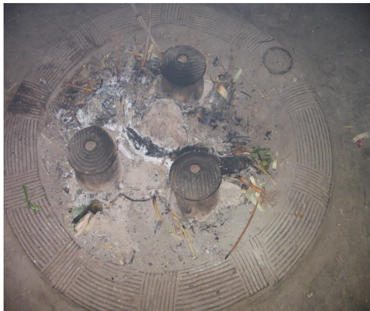
Photo 6.1: Three-stone fire place with interlocking semi-circular blocks making a complete circle and three pot stands in the middle, Haisie (a rural village near Hosaena town)
